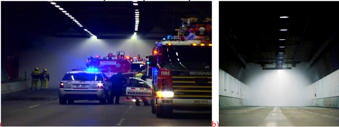
*Figure 4 a) A 'wall of smoke' on the edge of a ventilation zone during the Burnley Tunnel fire incident and b) deluge operation within the Clem Jones Tunnel (CLEM7) tunnel.*
